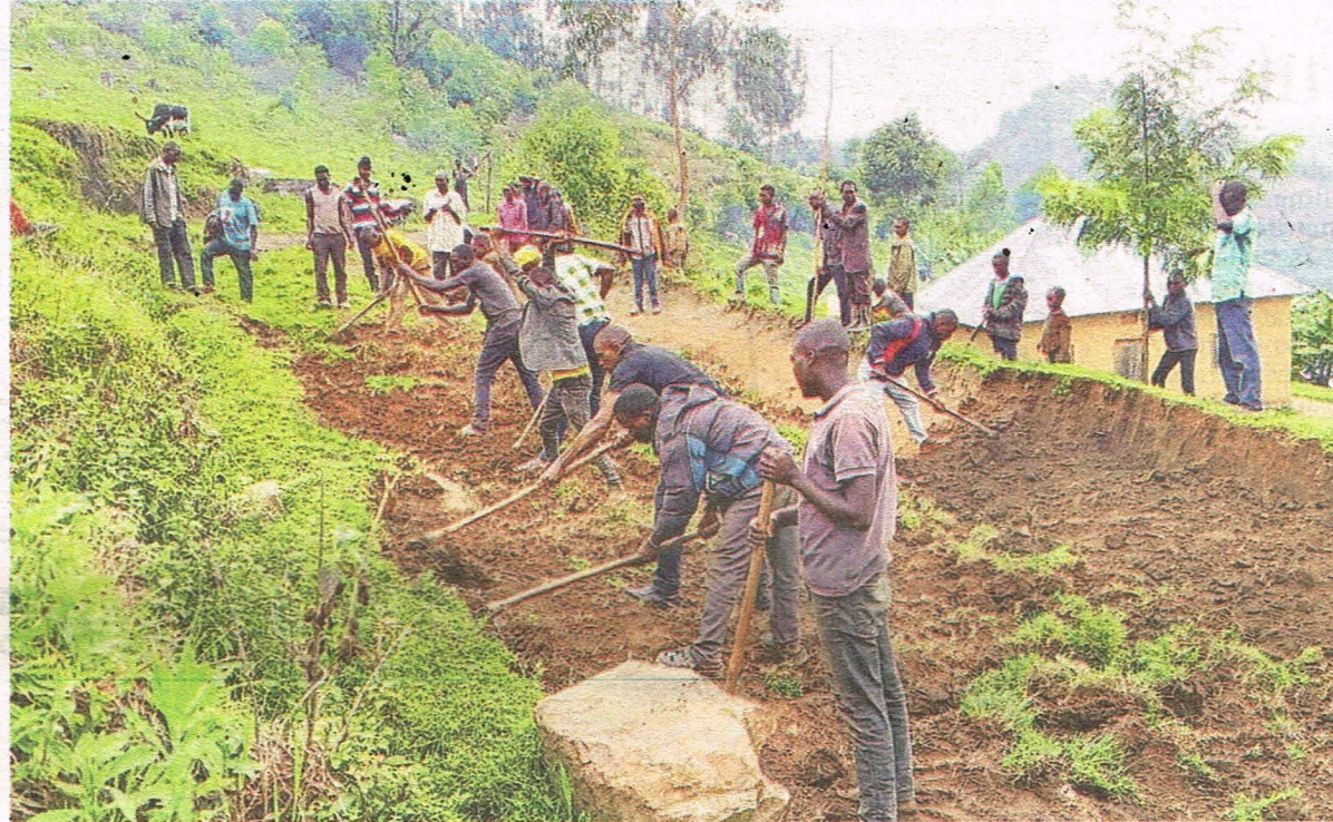
Residents dig a community access road in Kayonza Cell, Kayonza Parish in Rubengye Sub-county, Buhweju District, on January 11. PHOTO/JULIUS BYAMUKAMA
